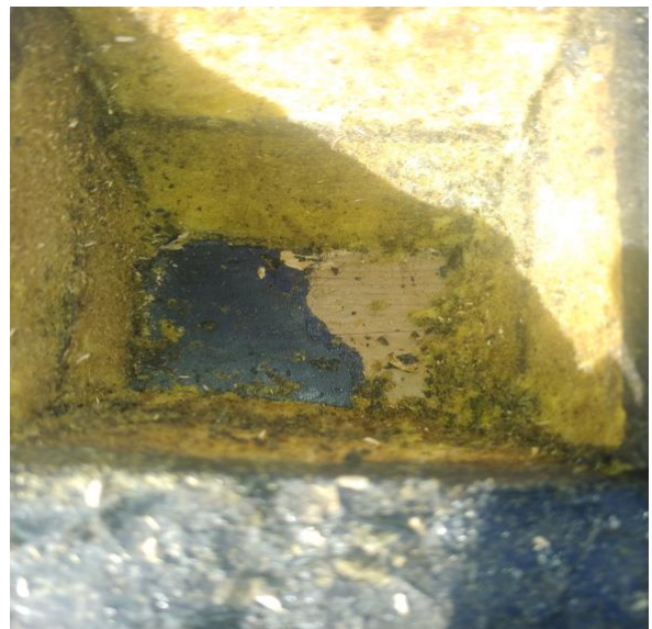
Photograph 4 – Roof 2.0 Cross-sectional view of Bitumen
