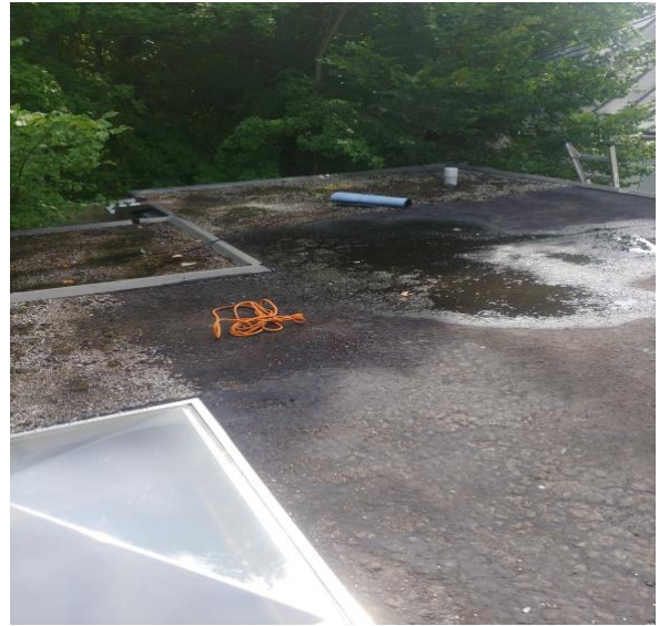
Photograph 2 – Canopy Classroom Roof
