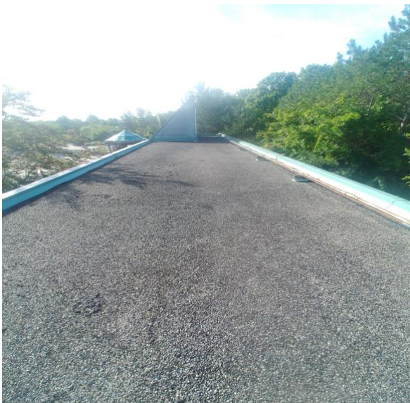
Photograph 3 – Education Building – Roof 2.1
